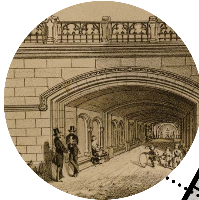
carriage road underpass
