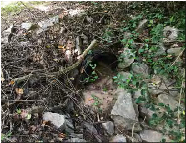
STORMWATER CULVERT CLOGGED WITH SEDIMENT
